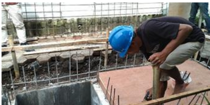
Constructing septic tank in Magelang.
