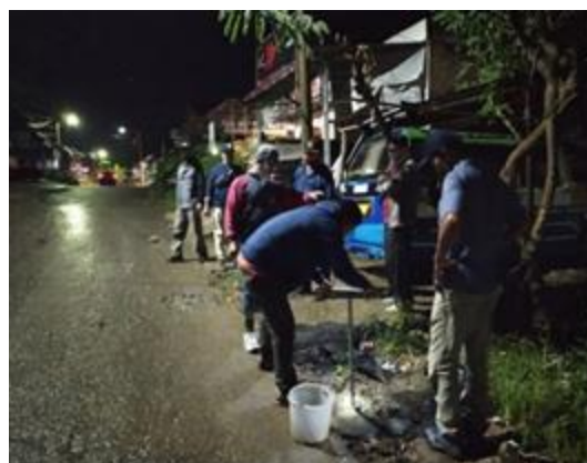
Preparation and Set DMA Location
