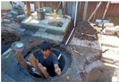
A mason is building a septic tank in Tunjungsekar village.
