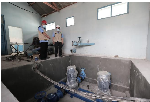
Photo caption: Two new pumps procured by Perumda Air Minum Kabupaten Sukoharjo to increase their energy efficiency
