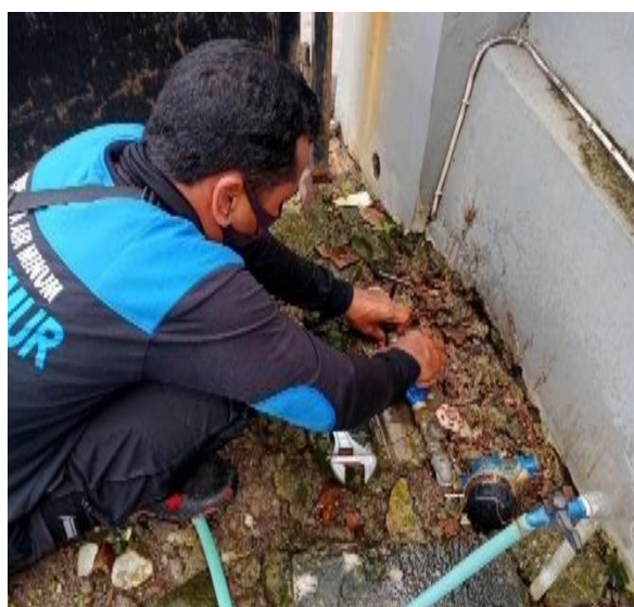
Photo caption: A staff of Perumda Air Minum Kabupaten Sukoharjo replacing a water meter
