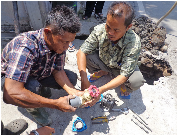
Technical training on Master Meter operation and maintenance (O&M) for CBO members in Surakarta, Central Java.
